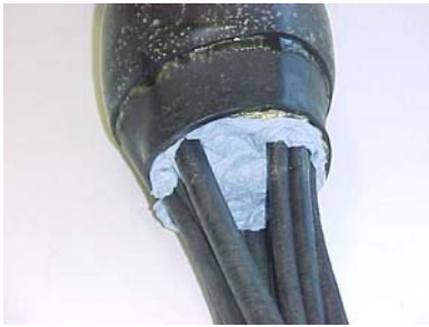
Fig.3. Closure 31J prepared for sealant
