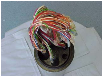
Fig. 1. Closure 31B prepared for sealant
