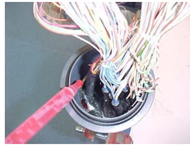
Fig.4. Closure 31J - Applying sealant.
