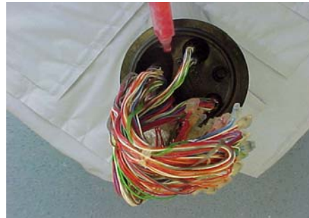
Fig. 2. Closure 31B - Applying Sealant.
