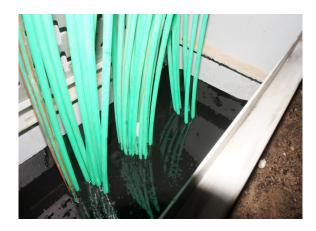
2 component sealant used to seal the base & ducts in Virgin Media's street cabinets.
