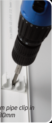
40x20mm makes it quick and easy to fit 10mm pipes
